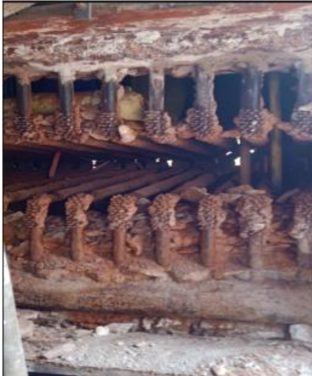
Before Single row bed coil replacement
