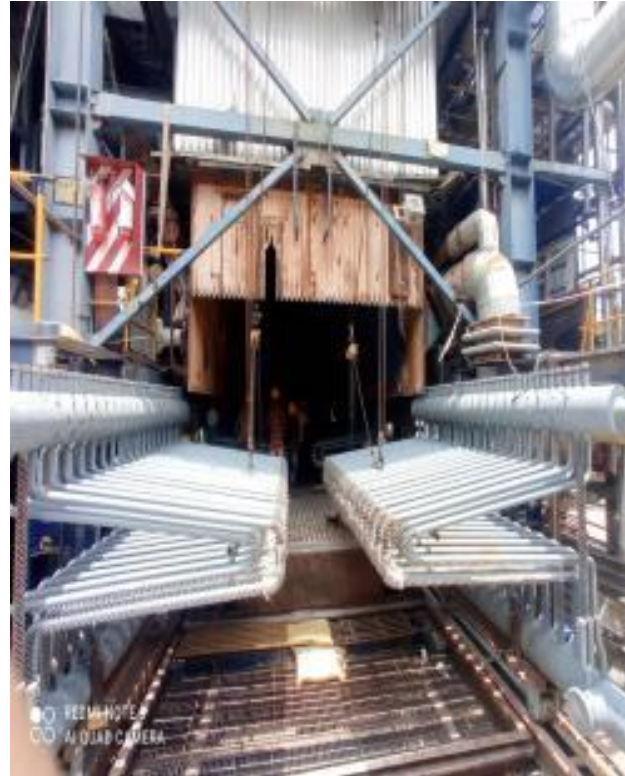
After Double row bed coil replacement
